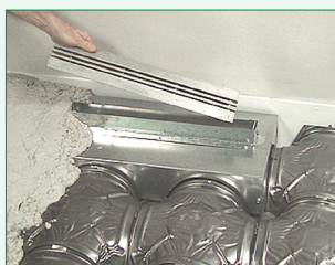
Flush registers accommodate carpeted and tiled floors.
