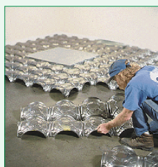
AIRFLOOR™ forms interlock to create a unified plenum.
