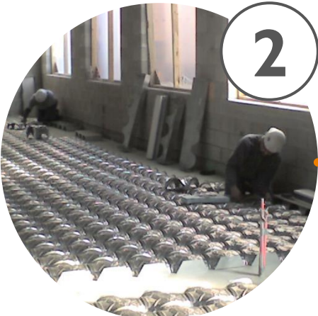
Airfloor™ forms laid down 1 person can install 1000sq.ft a day
