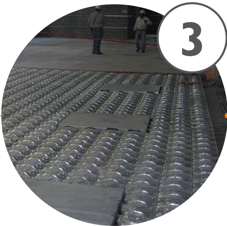
Airfloor™ splash boxes and ductwork installed
