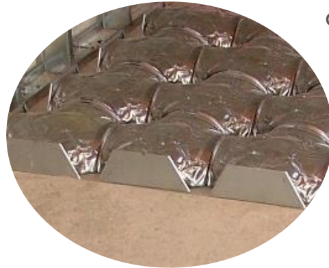
Form Closer & Divider Closer to seal off void formers for concrete pour and divider to direct airflow within Airfloor™ void
