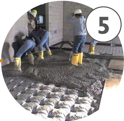
Topping slab poured
