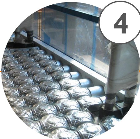
Airfloor™ form extensions and floor connectors installed
